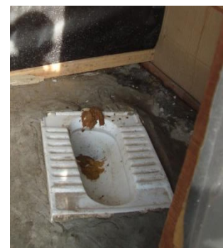
Fig.5. Toilet at Sunjwan
